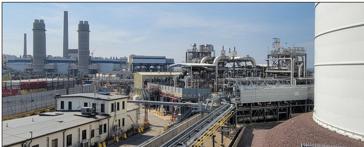
Figure 16. Mystic Generating Station (left), vaporization equipment (center), LNG storage tank (right)
