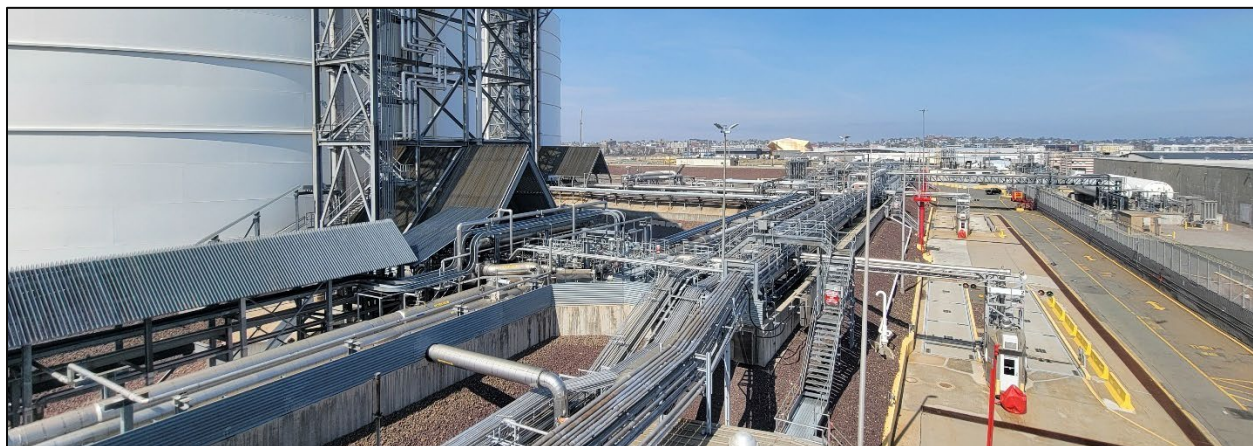
Figure 15. Truck loading bays at EMT (right).
