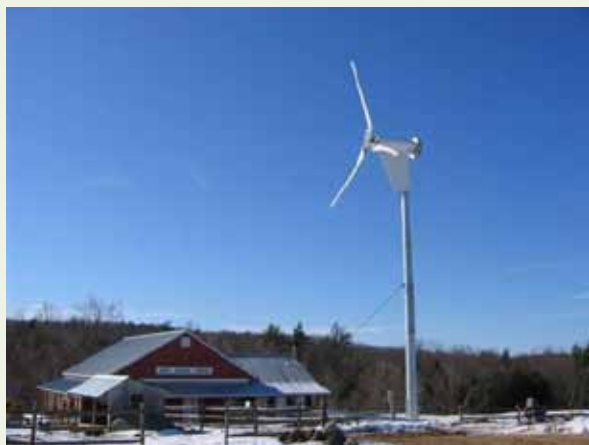
In 2009, the Department contributed $25,000 towards the cost of a 15KW wind turbine for Red Apple Farm. At an elevation of 1,250 feet, Red Apple Farm is one of the highest commercial orchards in New England. A 15KW system is expected to produce roughly 19,100kWh of electricity on an annual basis, representing 77% of Red Apple Farm's current electricity usage.
